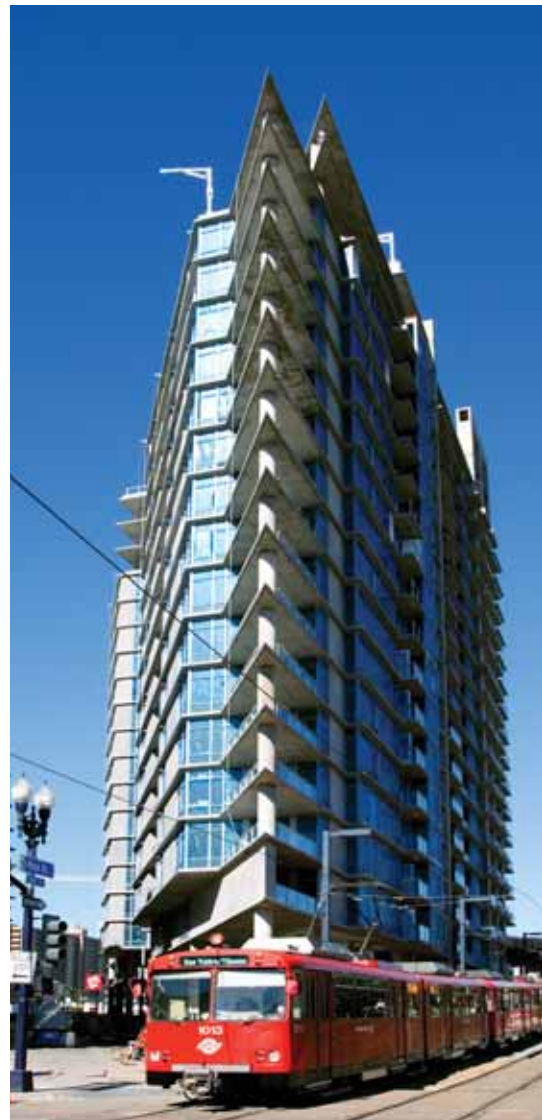
Smart Corner, a housing project that incorporated transit and many more sustainable elements in its design.
